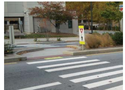
Refuge islands provide a place for pedestrians to wait out on-coming traffic within wider right-of-ways Image: www.peopleforbikes.org /Lyubov Zuyeva
